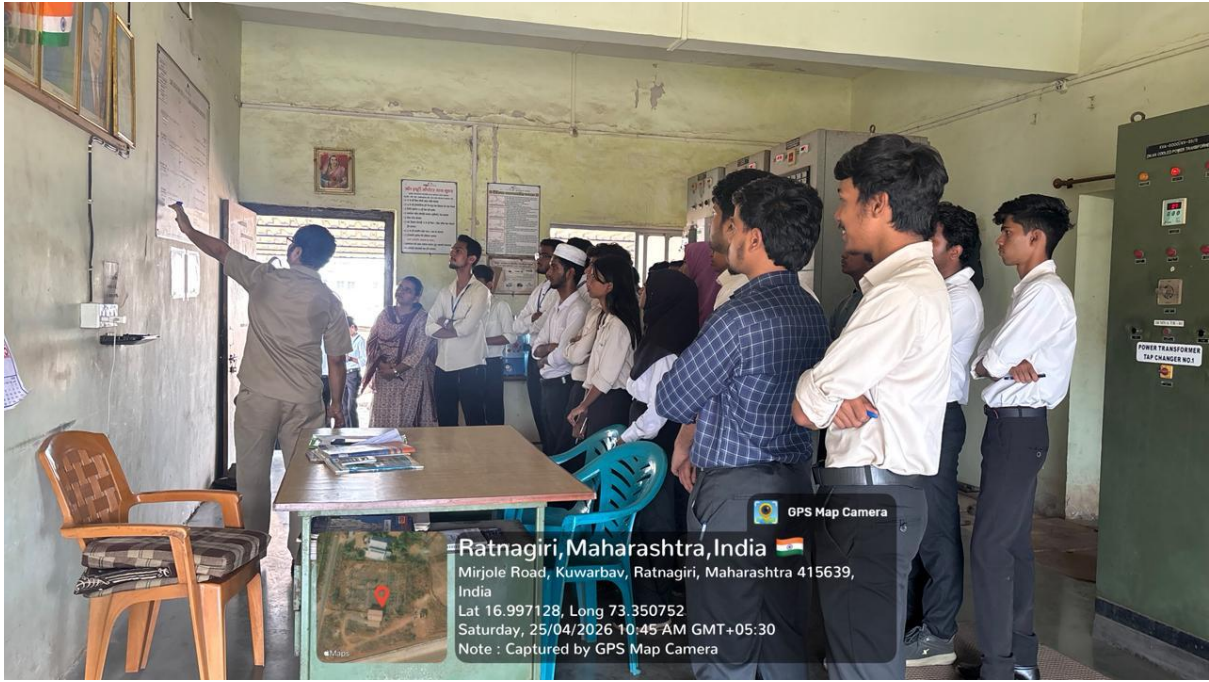
Mr. Malusthe explaining the Single Line Diagram and Control Panels of Substation
