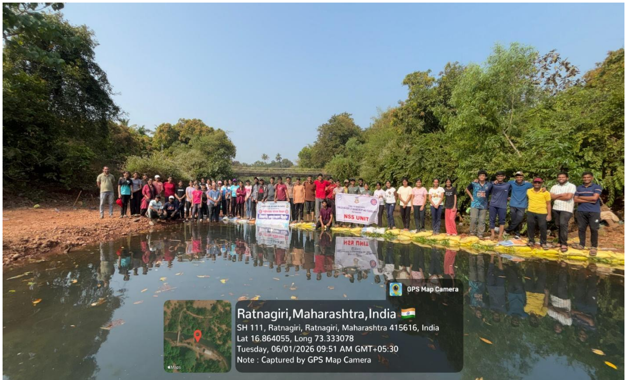
Constructing Progress, together!!
