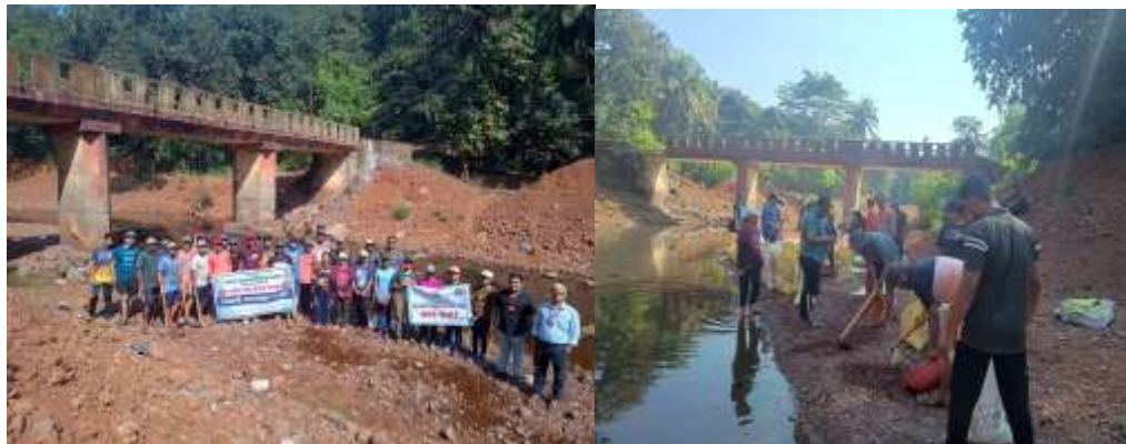
Construction of Dam by Volunteers
