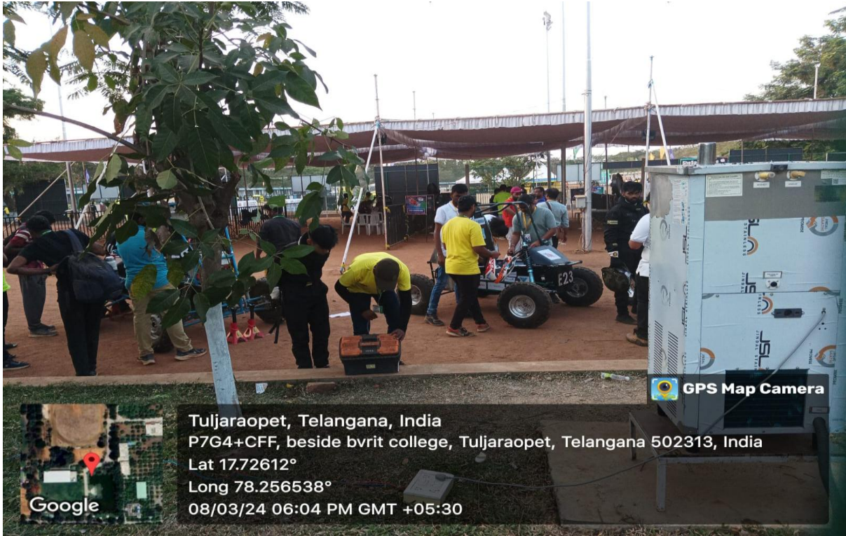
Team Matadors clearing the Mechanical and overall Build quality inspection
