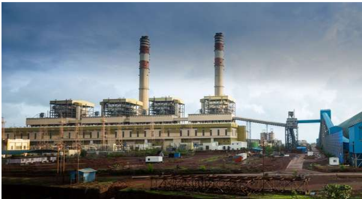
JSW power plant
